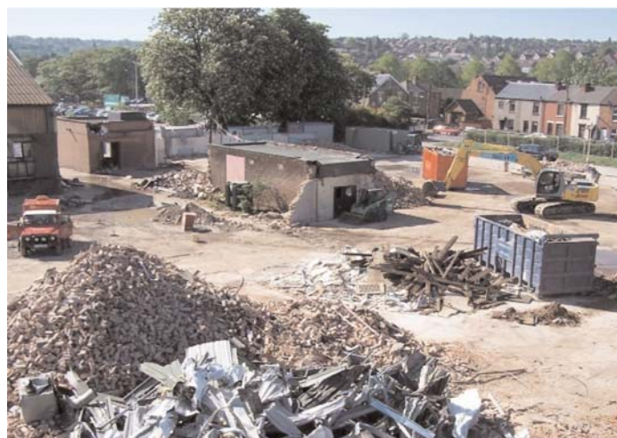
Figure 4: Demolition in progress
